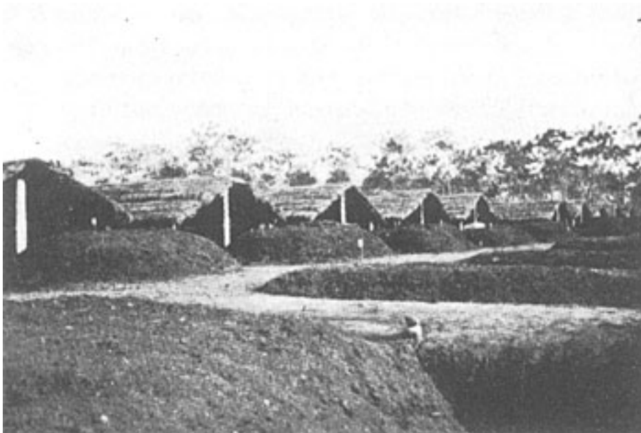
Covered and uncovered pits.
