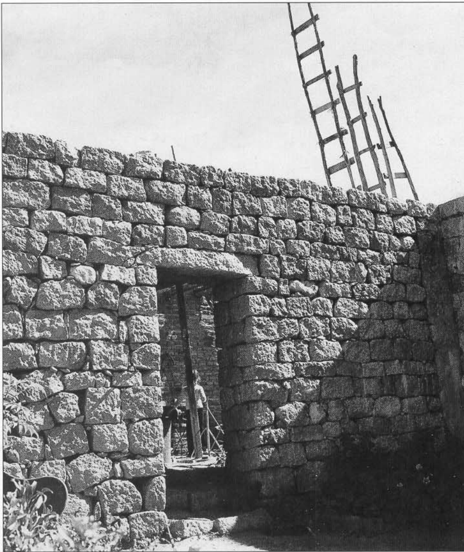
Figure 6: "Dry-wall construction with squared granite boulders in Argentina"
