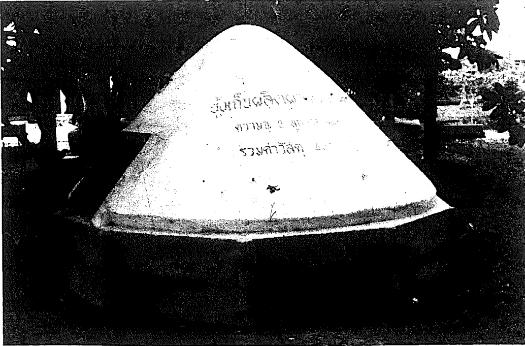
Figure G1: Completed cement mortar bin
