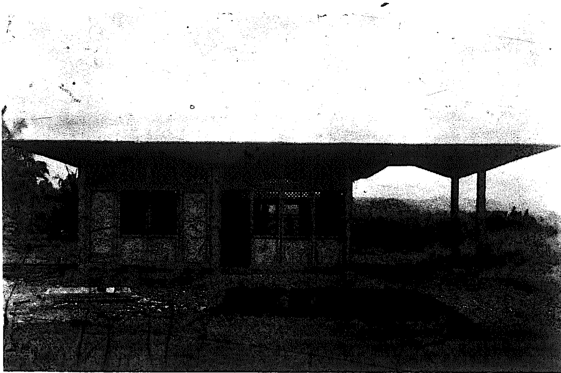
Figure E3: Elevation of prototype ferrocement house
