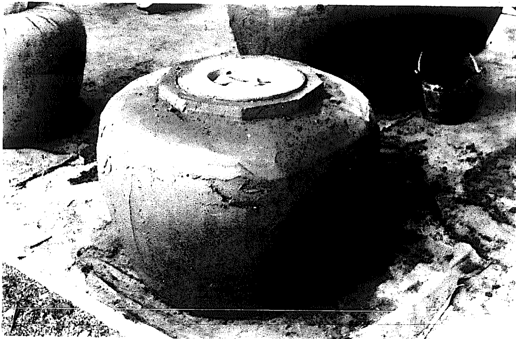
Figure K8: The first layer of cement mortar is applied from the bottom to the top with a thickness of about 0.5 cm.
