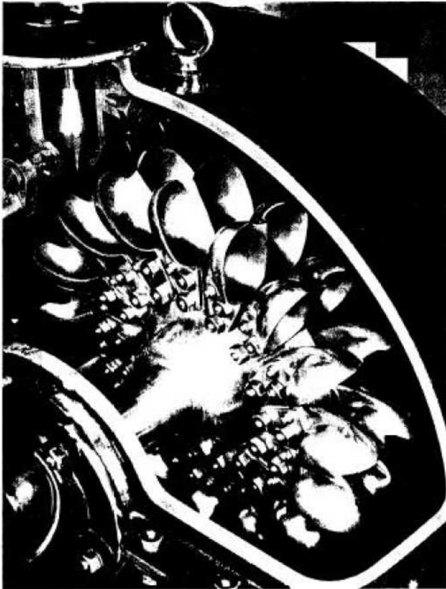
15 Model of a Pelton wheel with nozzle regulator.
