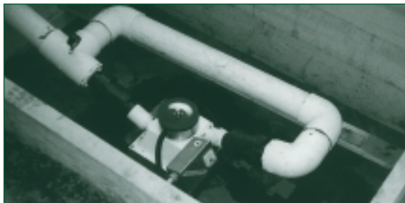
Stream Engine Installation
