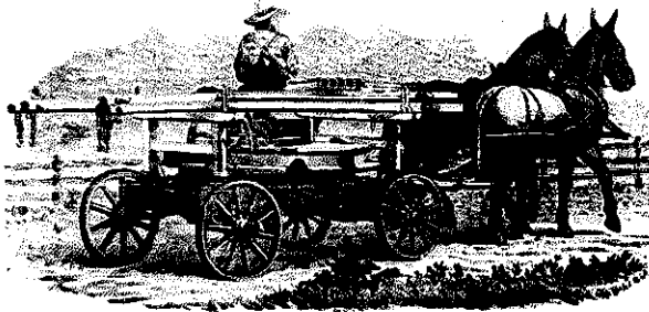
During the 1840s, implement manufacturers began building portable horse-powered sweeps. Portable sweeps gave the farmer greater flexibility at threshing time. These sweeps were characteristic of those built during the late nineteenth century.
