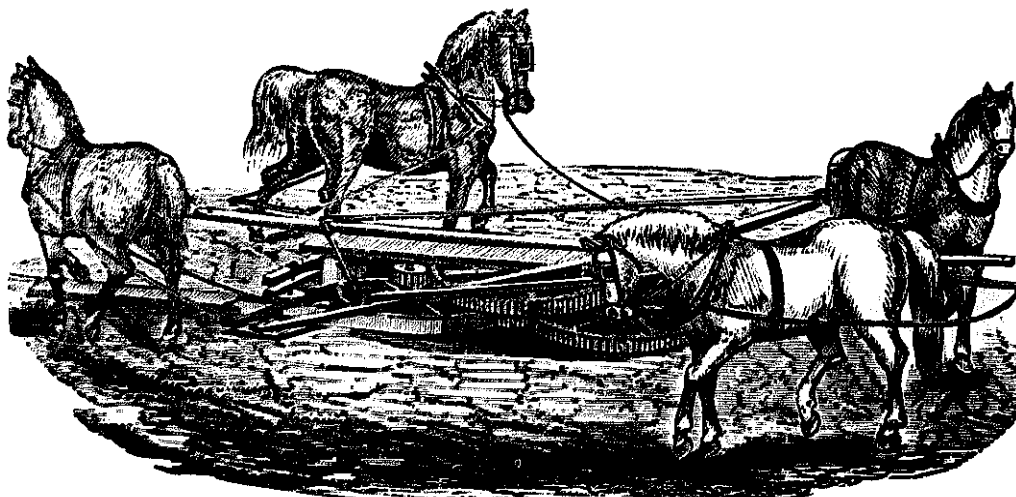
Above: On small farms, the treadmill most commonly powered the threshing machine. Power transferred from the treadmill to the threshing machine by the belt in the center of the illustration. (Smithsonian Institution.)
