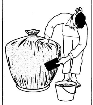
3. When full, tie the top sacking and form into a jar shape by tapping with a block of wood. Spray with water before plastering.
